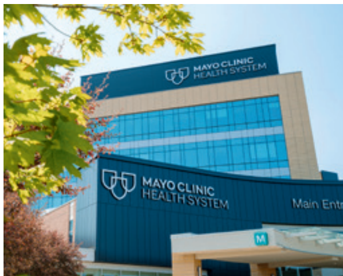
Top: The new six-level Mayo Clinic Health System hospital in La Crosse, Wisconsin.
